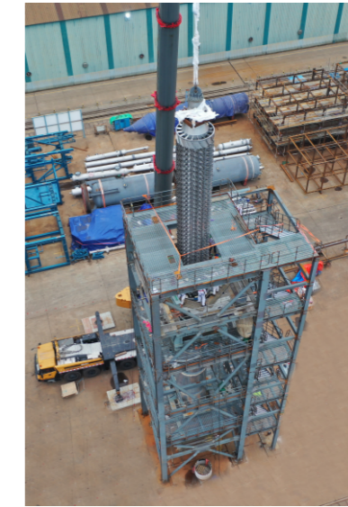
安装调试 Installation and debugging
